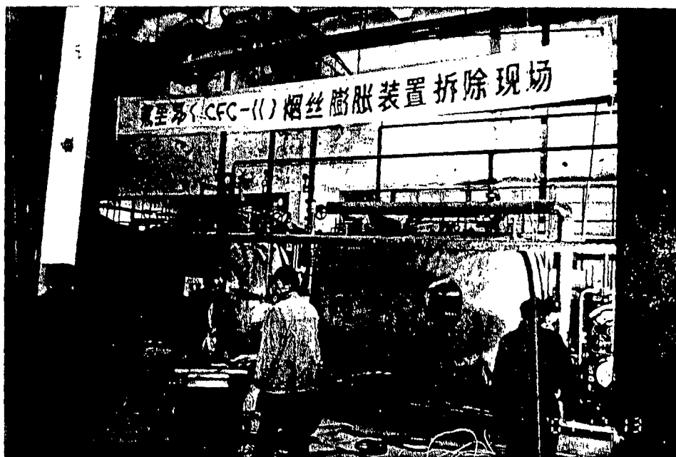
The CFC-11 equipment locale for dismantle
