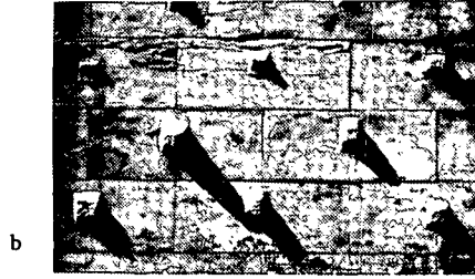
3.10 Random coursed and isodomic masonry, Mycenae and Athens
