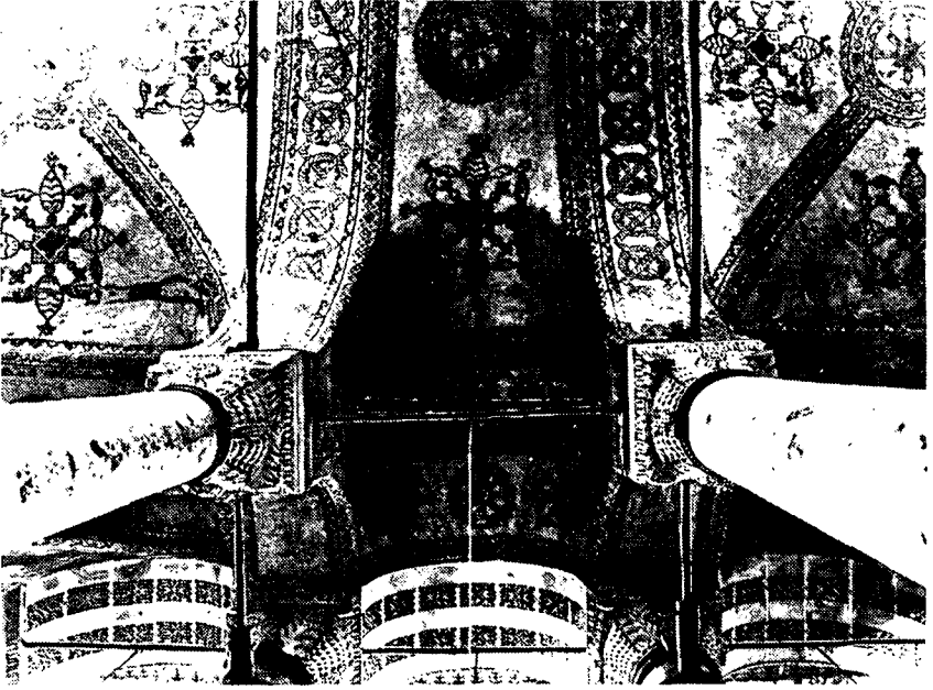
3.49 Vaults and ties, south aisle, Hagia Sophia, Istanbul
