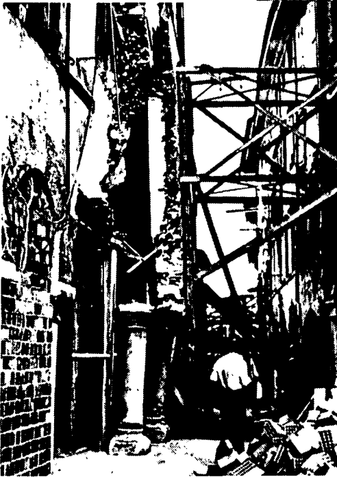
3.90 Damaged building, Venzone
