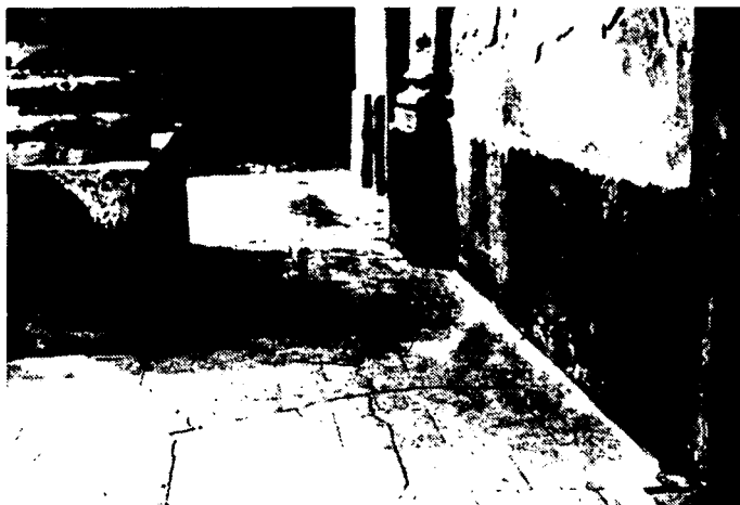
12.2 Cracks in the paving of the main entrance
