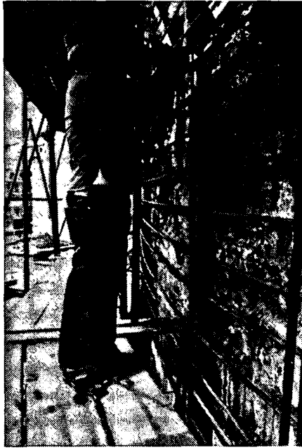
8.6 Prestressing of temporary external steel rings
