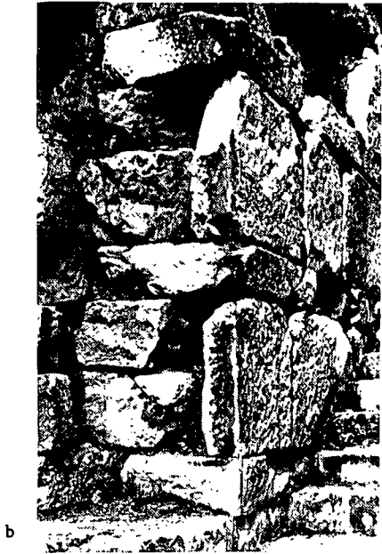
3.11 Pseudisodomic masonry, Delphi and Ephesus
