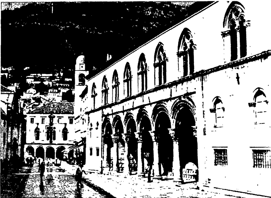
15.1 General view from the southwest
