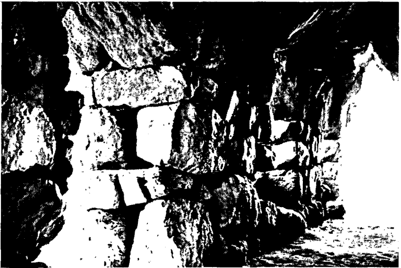
3.7 Fortress wall of large roughly dressed un-mortared blocks, Tiryns
