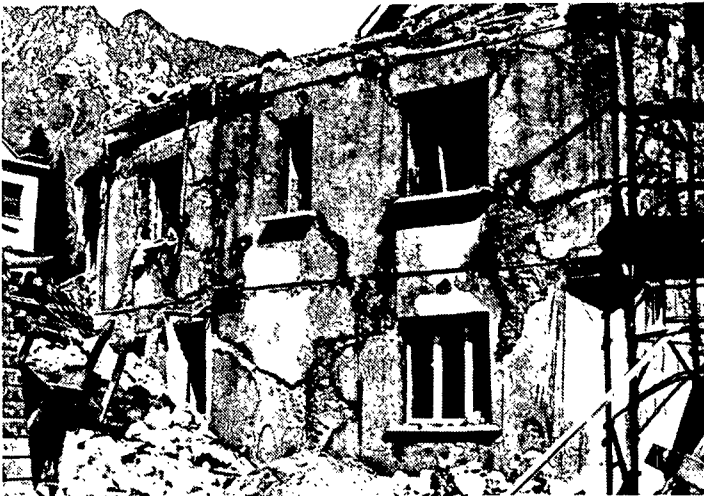
18.18 Building in Lusevera after the September 1976 earthquakes
