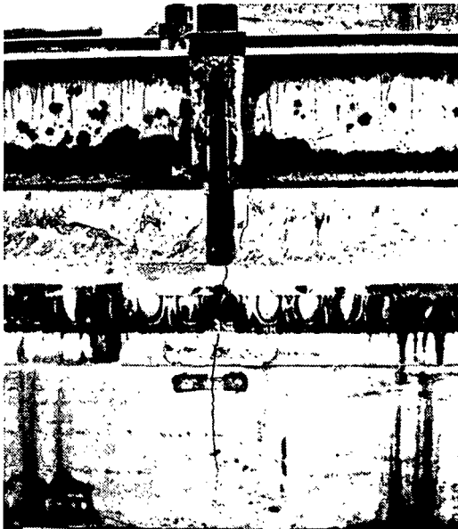
7.10 Fracture of an architrave of the north porch due to rusting of hangers
