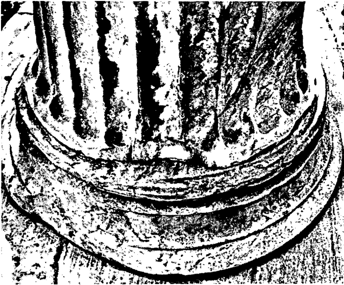
7.12 Fractures at the foot of a column, east porch
