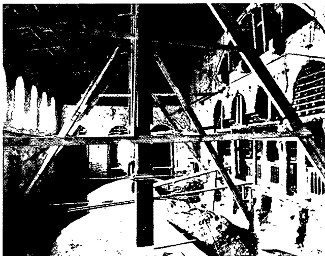
5.26 Fills removed over side aisle and narthex vaults, Hagia Sophia, Thessaloniki
