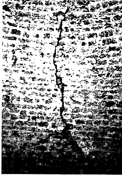
11.3 Cracking of the dome
