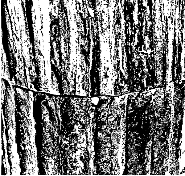
7.11 Fractures on the edges of column drums, east porch
