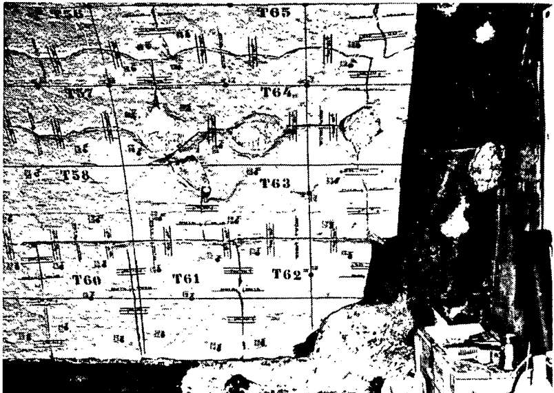
5.7 Preparation for removal of mosaics, Rotunda, Thessaloniki
