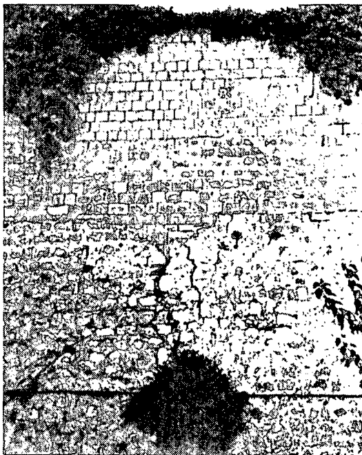
5.10 Cracking of a wall after repair, Castle of Heraklion
