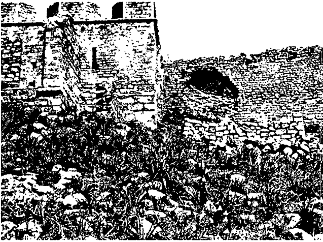
14.2 Damage initiated by gunfire, Castle of Acrocorinth
