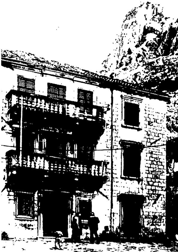
16.1 View of the main frontage
