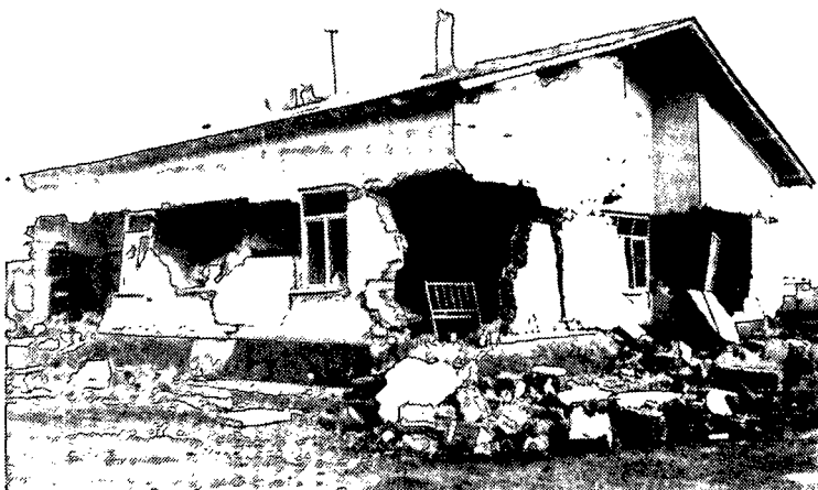
Fig.3.9 - Caldiran,1976 Earthquake (Turkey):Partial collapse of window piers and corner zone; brick masonry public building
