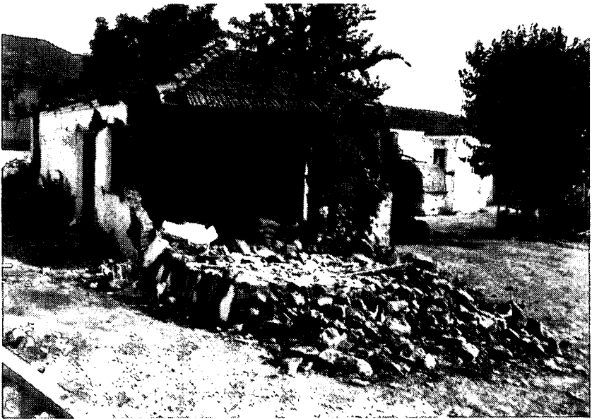
Fig.3.4 - Thessaloniki,1978 Earthquake (Greece): Overturning of a head wall; rural stone-masonry dwelling house
