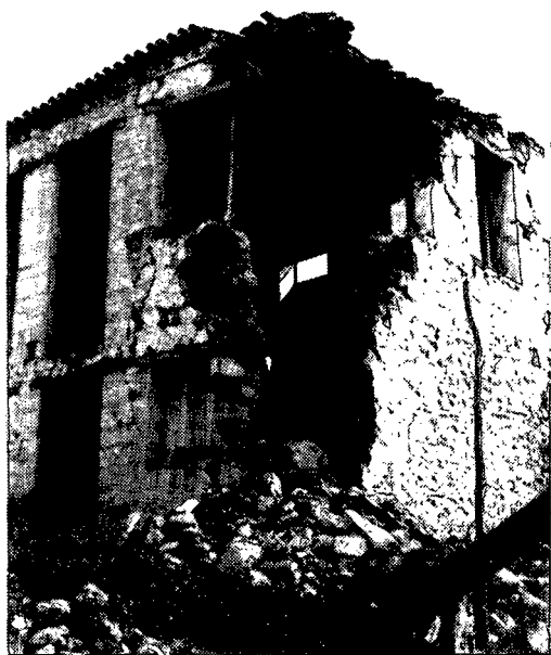
Fig.3.10 - Corinth,1981 Earthquakes (Greece):Partial collapse of walls and corner zone;stone-masonry rural dwelling house
