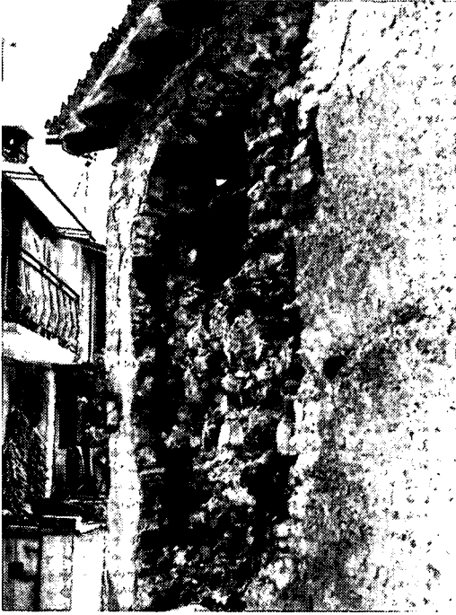
Fig.3.11 - Friuli,1976 Earthquake (Yugoslav territory):Disintegration of a stone-masonry wall;stone-masonry dwelling house
