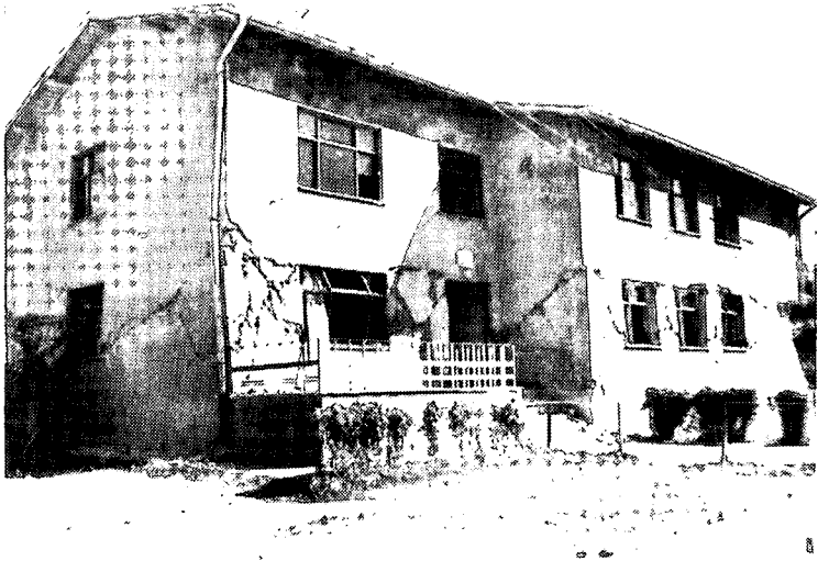
Fig.3.7 - Lice,1975 Earthquake (Turkey): Typical diagonal cracks in window piers; brick masonry public building
