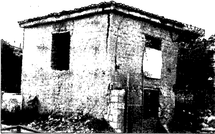
Fig.3.2 - Magnessia,1980 Earthquake (Greece): Vertical cracks at the joints of walls; rural stone-masonry dwelling house
