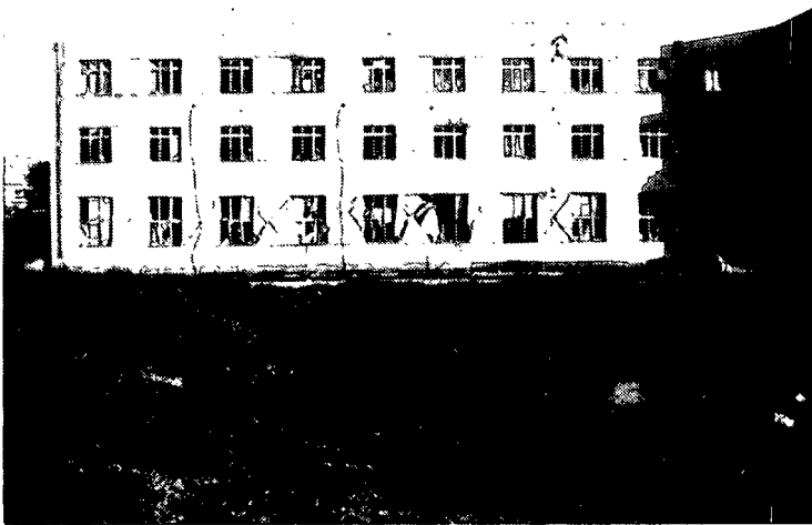
Fig.3.6 - Montenegro,1979 Earthquake (Yugoslavia):Typical diagonal cracks in window piers; brick masonry building
