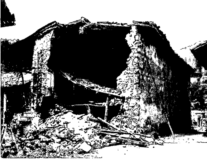
Fig.3.5 - Friuli,1979 Earthquake (Yugoslav territory): Overturning of a head wall; rural stone-masonry house
