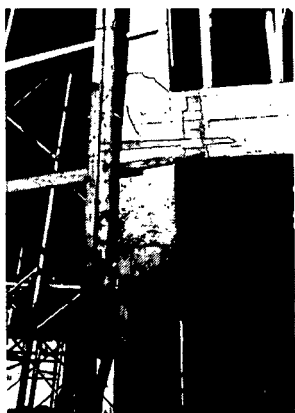
(a) Very poor concrete at upper end of column
