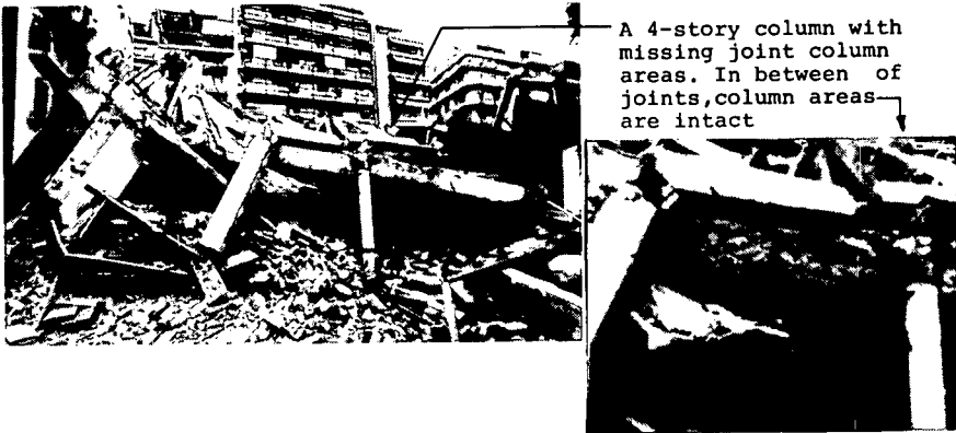
(e) Insufficient and improper structural joint reinforcement
