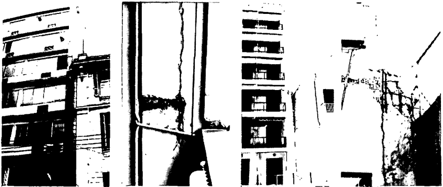
Exterior view Interior view General view Detail (a) Structures with different heights
