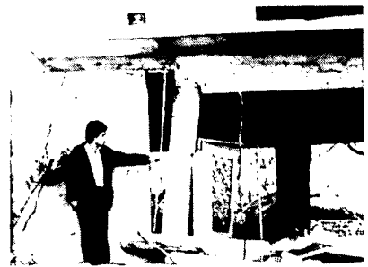
Fig.2.13 Causes of overstress. Problems due to torsional motion [22]
