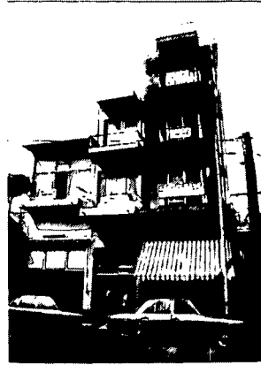
c) view of severe case
