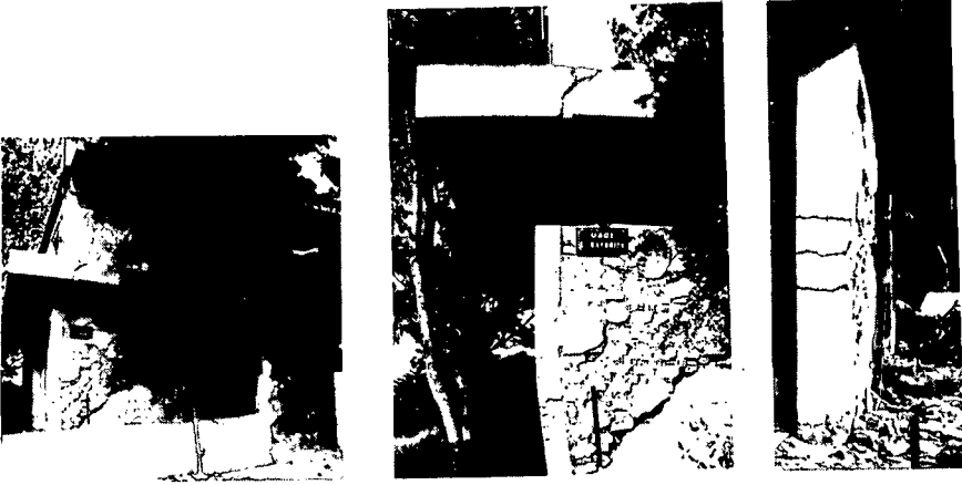
(c) Mid-height column damage due to interaction
