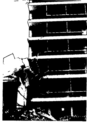
Fig. 2.11 Causes of overstress. Structure to structure interaction [22] (continued)
