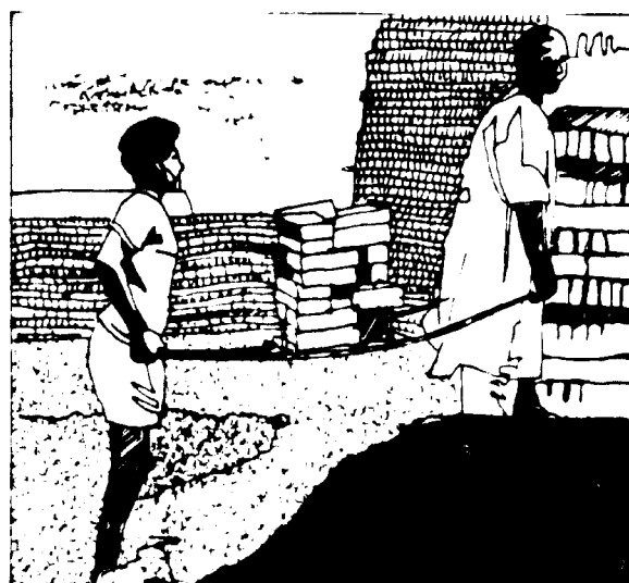
Two men carry dry bricks up to the clamp for setting.
