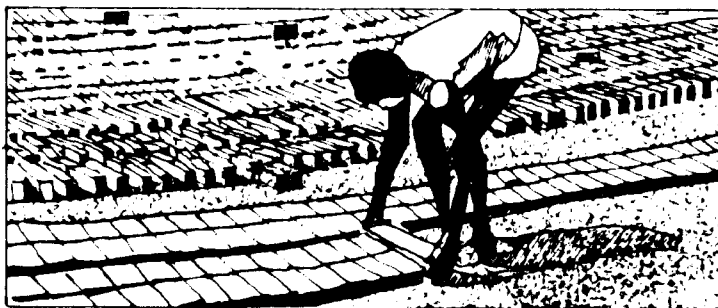
Brick carrier takes bricks in mould to the drying ground, (fibrous material in the clay prevents cracking).
