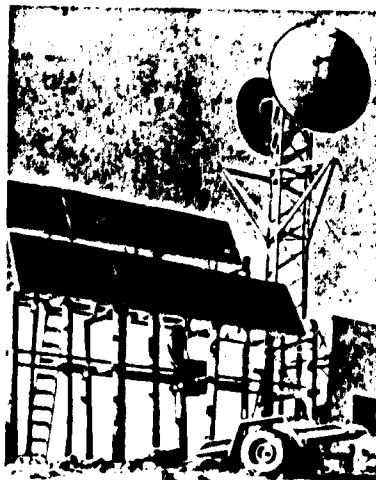
Solar Power Corporation's generators provide economical operating power for unmanned communications repeater stations.
