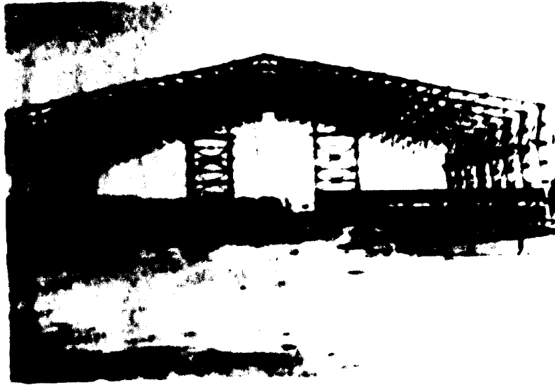
Coach house in Libya Constructed by a Greek structural steelwork Company with prefabricated in factory elements Span : 40 m Length: 80 m
