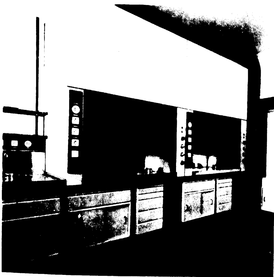
Fig. II Fume cupboards with baffle and by-pass, on concrete cantilevers, bench top covered with stainless steel, carcasses on casters
