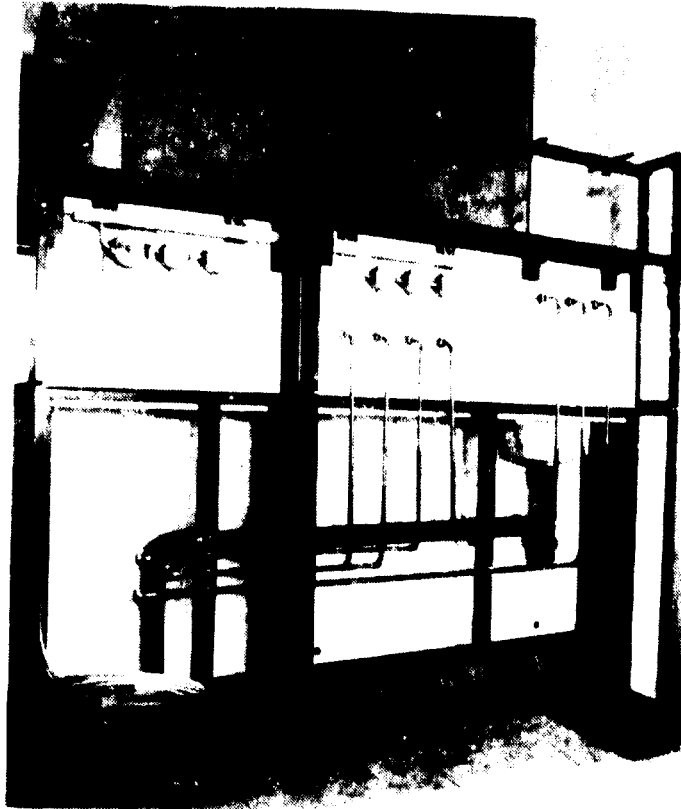
Fig. VII Prefabricated piping system made from copper tubing and plastic pipes
