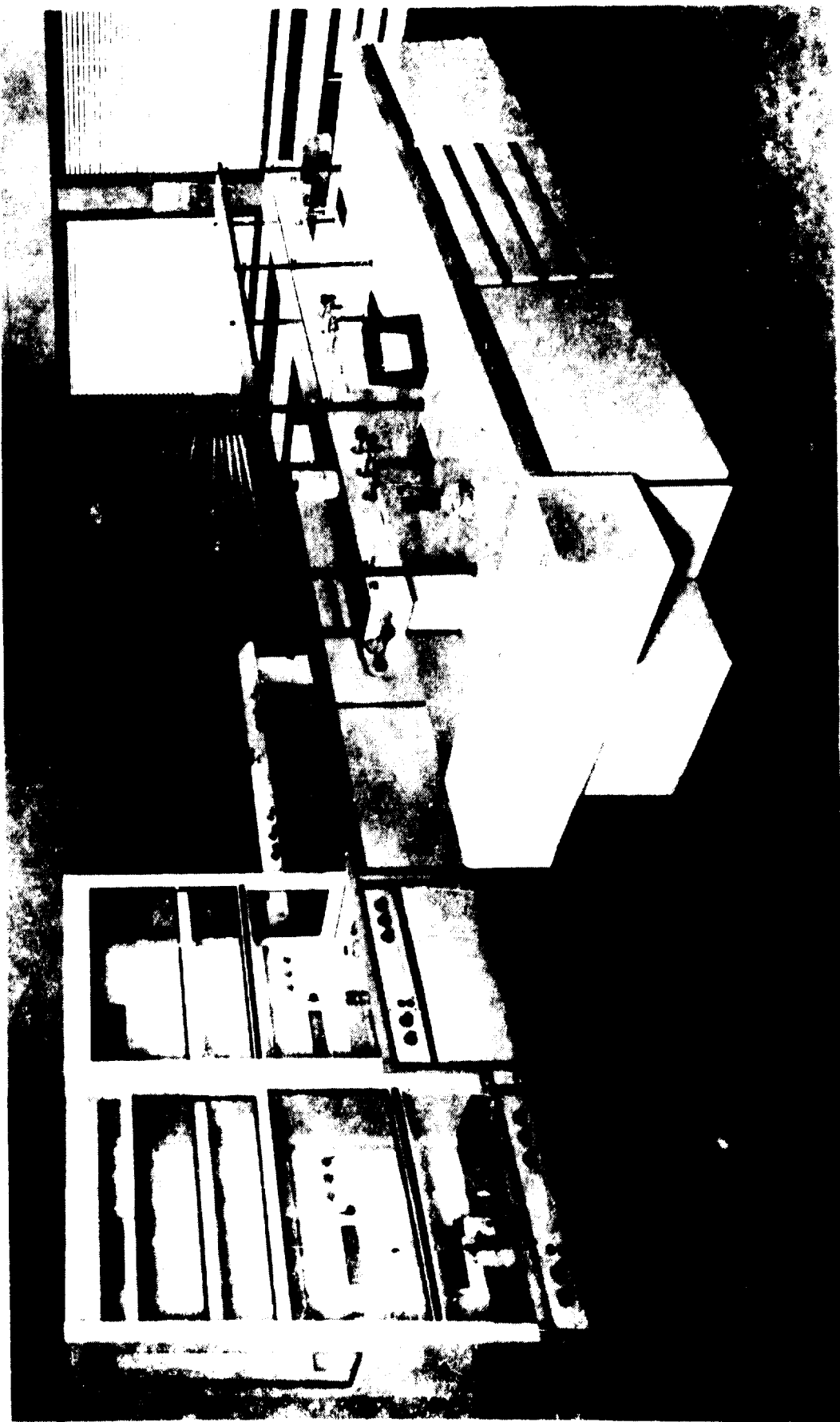
Fig. 7. Island and wall benches, with service shelves, ceramic sink unit, steel frame for carrying the bench tops and the carcasses made of plastic-laminated timbers. Staircase and I-w-bench frame not shown.
