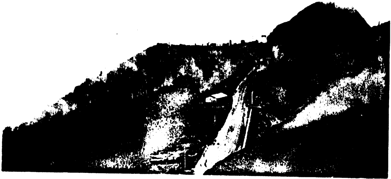
Nimba-Footwall road leading to Main Orebody and mine workshop
