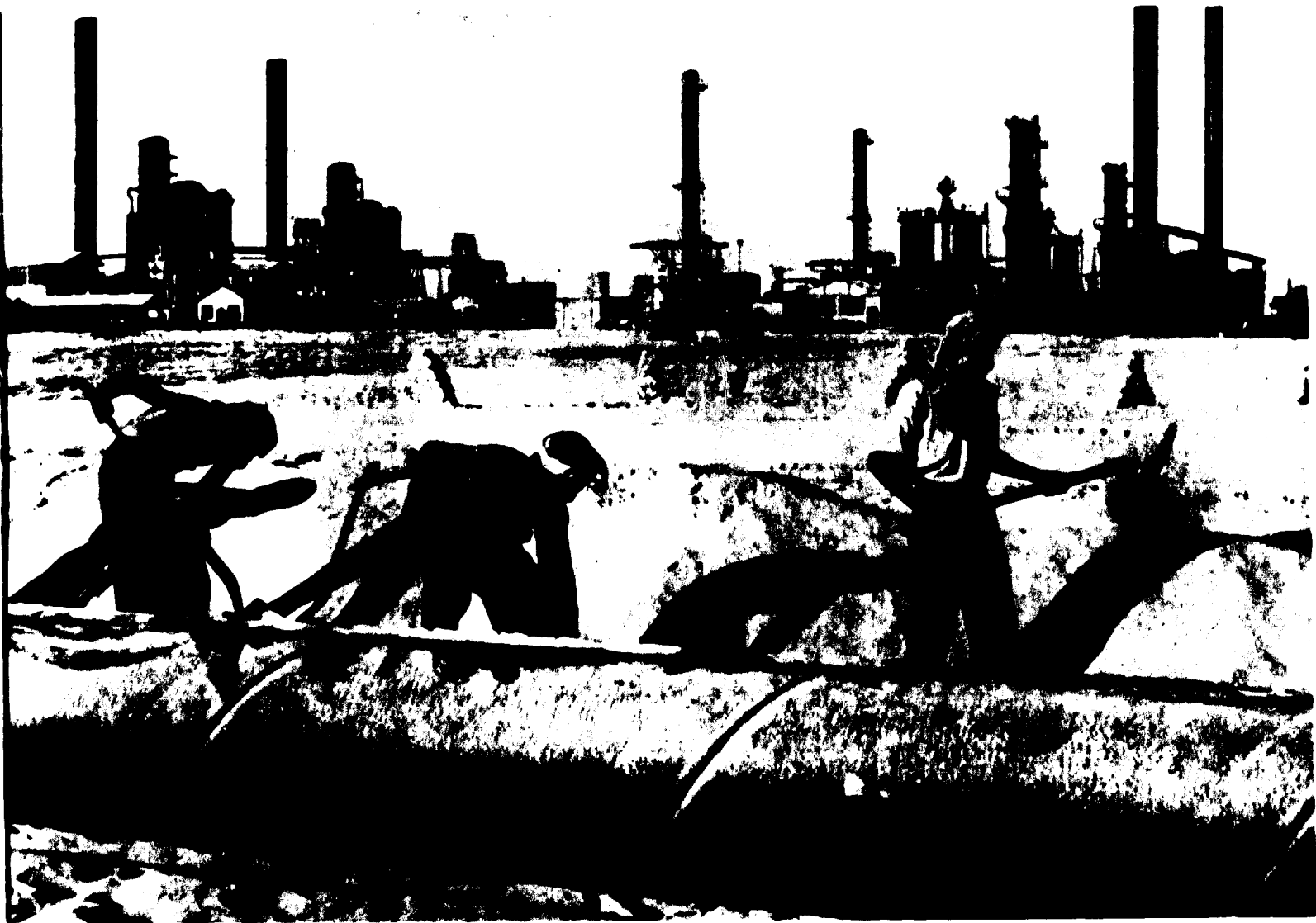
Laying a pipeline near the Ras Tanura refinery at Al Hasa, Saudi Arabia
