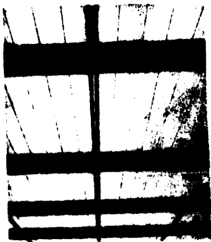
Fig.21. A roof of reinforced cell concrete plates.
