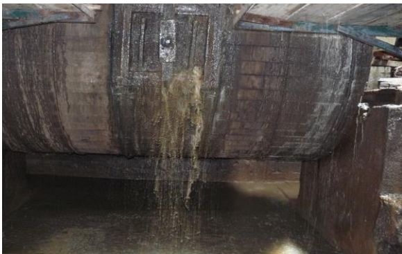
Photo 1; Old leaking drums before RECP
