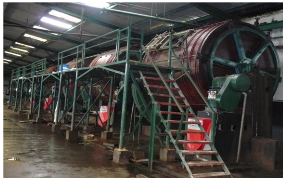
Photo 2; New installed drums of RECP
