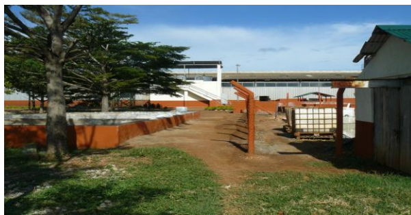
Photo 4; WWTP after RECP Implementation
