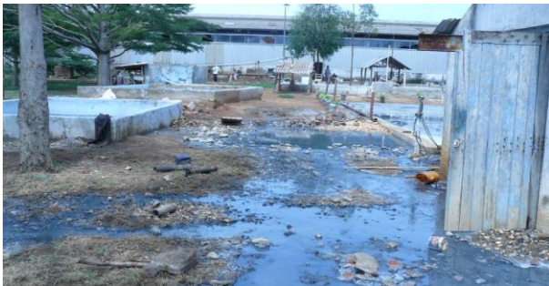
Photo 3; WWTP Before RECP
