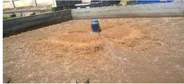
Waste water foaming has been eliminated after RECP implementation
