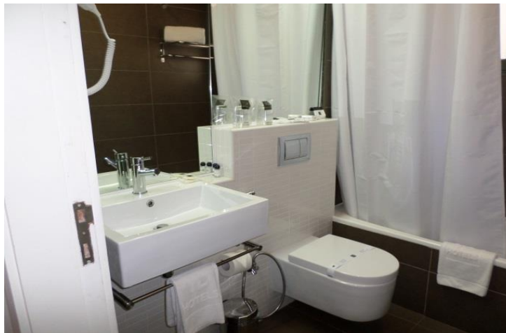
Figure 6: Dual flush tanks and water flow regulators in taps and shower caps
