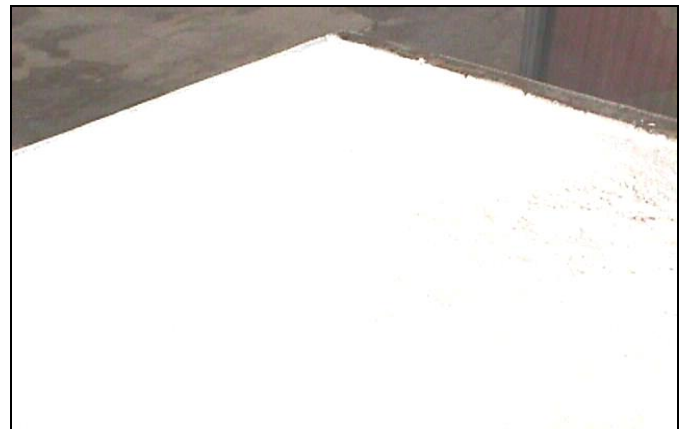
After installation of view of the Antisolar Coated Roof
