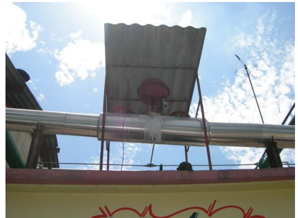
Figure 2. Insulation the steam distribution line
