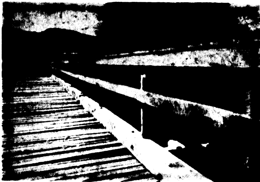
19. Detail of completed railing
