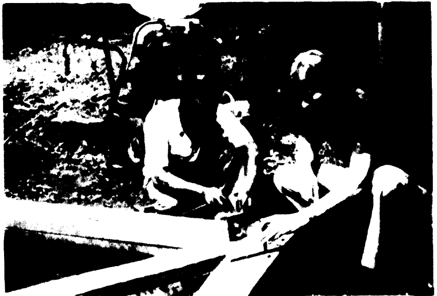
5. Bolting metal gusset plate on apex of element
