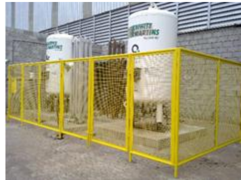
Figure 4: After Cleaner Production: Gas Station
