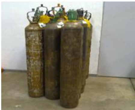
Figure 3: Before Cleaner Production: Gas supply by cylinders and bottles
