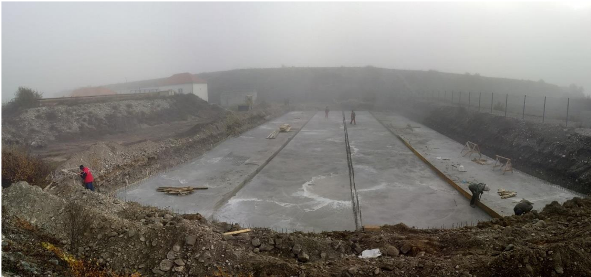
Figure 39: Finishing concrete works for trenches and bottom plates of SDRB
