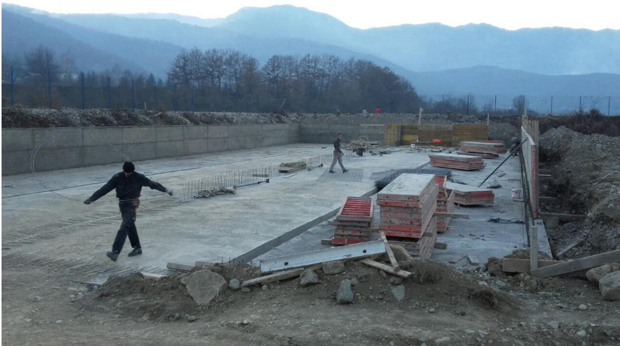
Figure 40: Preparation of side walls formwork
