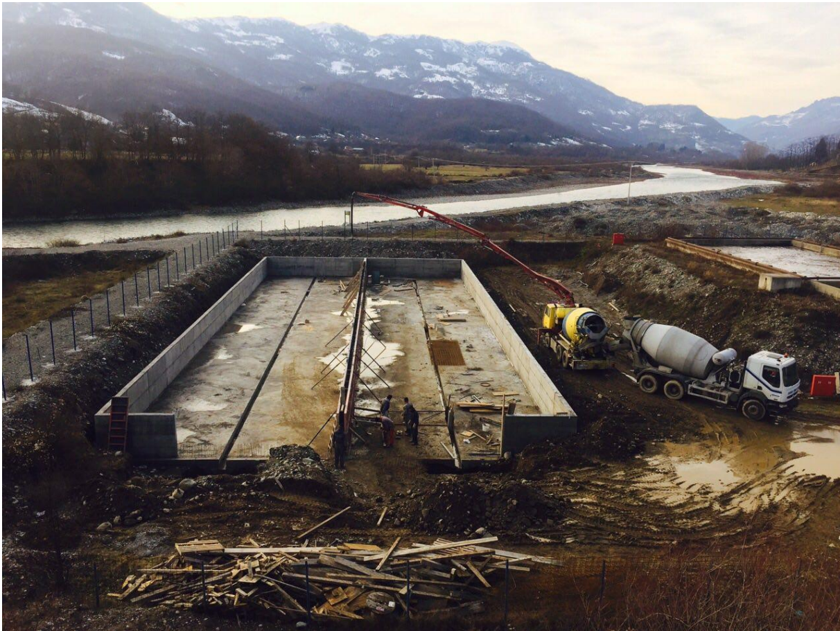
Figure 41: Concrete works on middle wall
