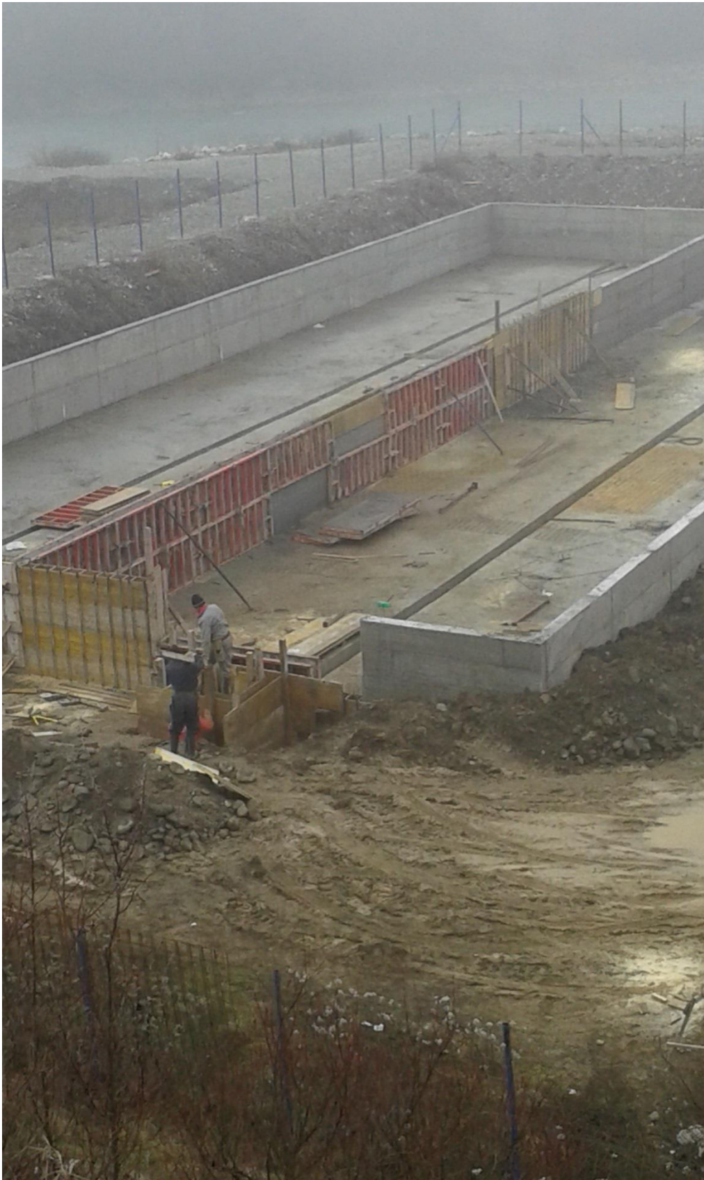
Figure 43: Formwork installation for seepage manholes.
