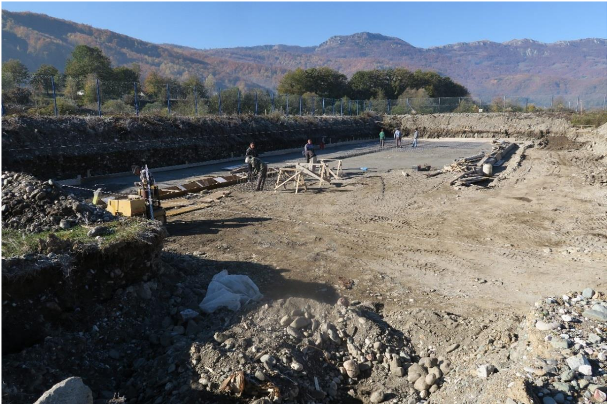
Figure 35: Lining concrete and reinforce steel placement for bottom plate of SDRB
