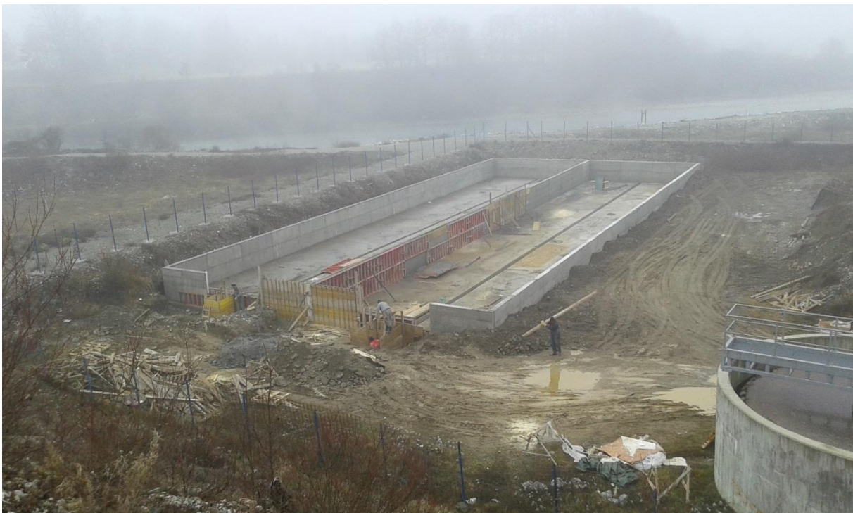
Figure 42: Closure of concrete works on walls
