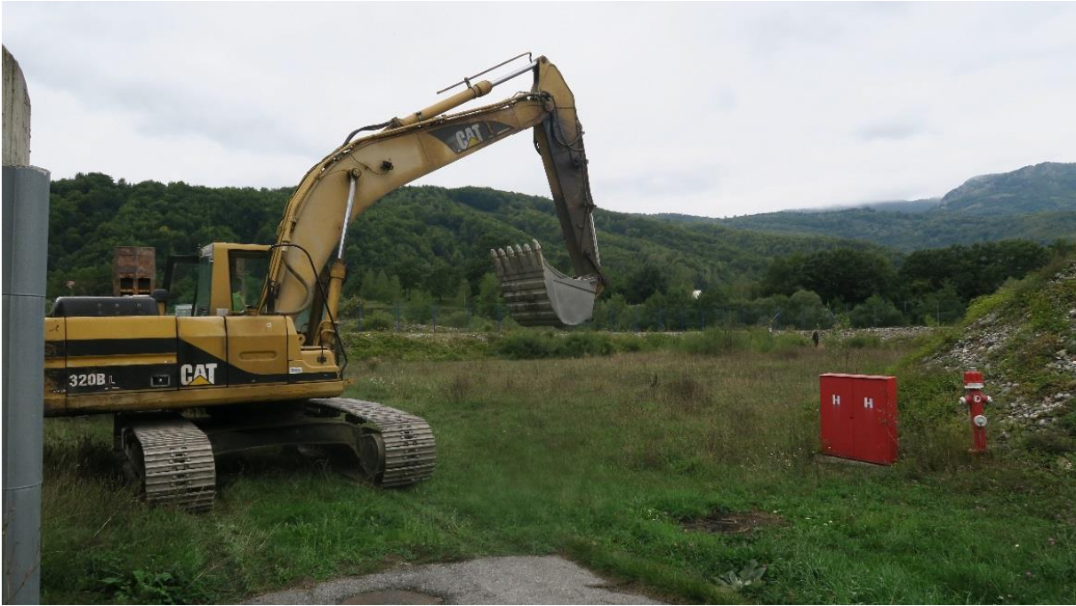
Figure 32: Excavator used for earthworks
