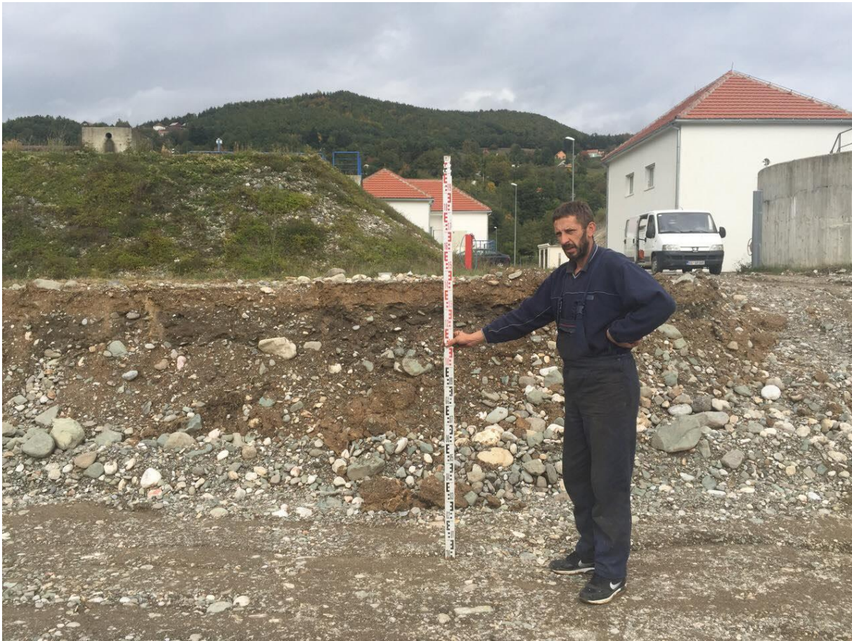
Figure 34: Depth of excavation
