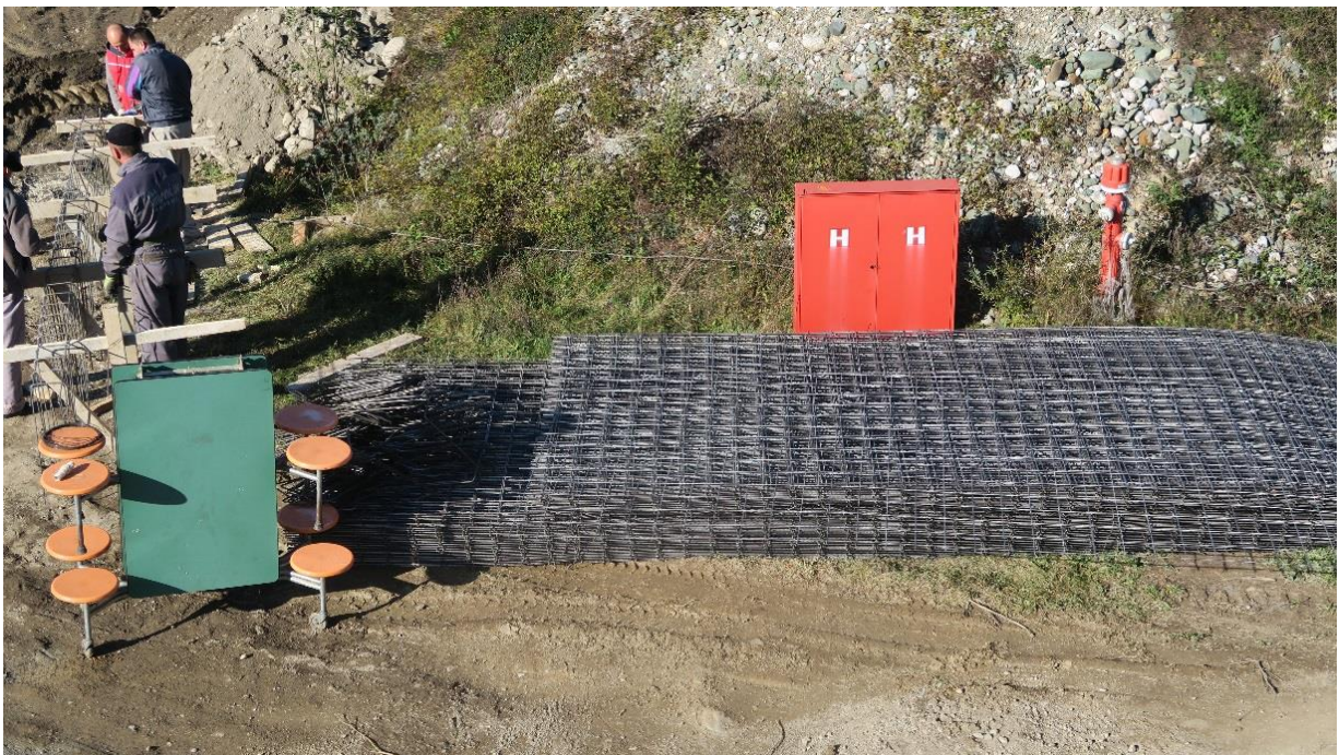
Figure 36: Material used for reinforcement
