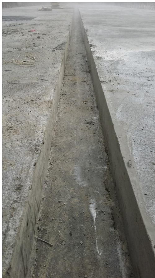
Figure 38: Detail of final trench concreting.
