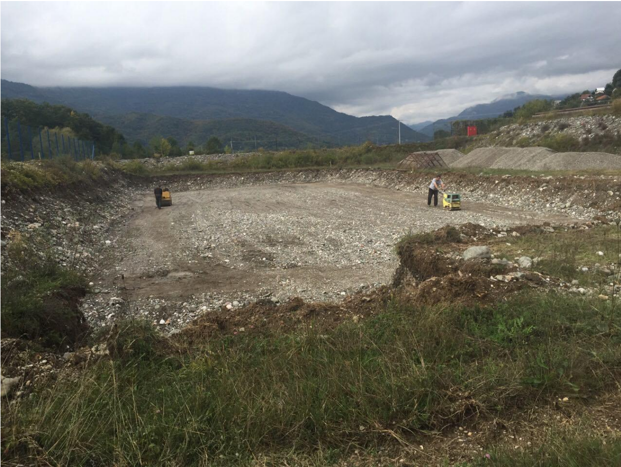
Figure 33: Compacting the tampon zone with tape vibrator
