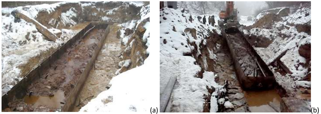
Figure 6: (a) Opening of emergency tanks, and (b) removal from excavated pit.
