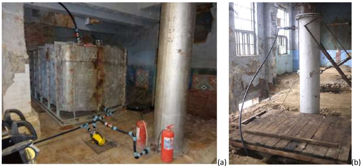
Figure 3: (a) Wastewater treatment and neutralization system, and (b) top of the active carbon absorption column
