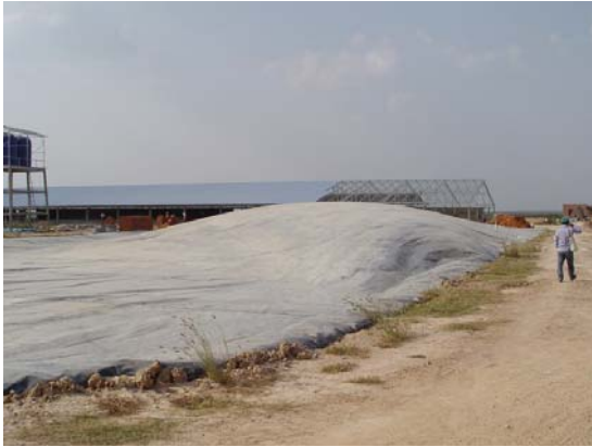
Figure 22: Kuch Sokha covered lagoon digester
