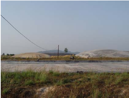
Figure 17: Covered lagoon digesters
