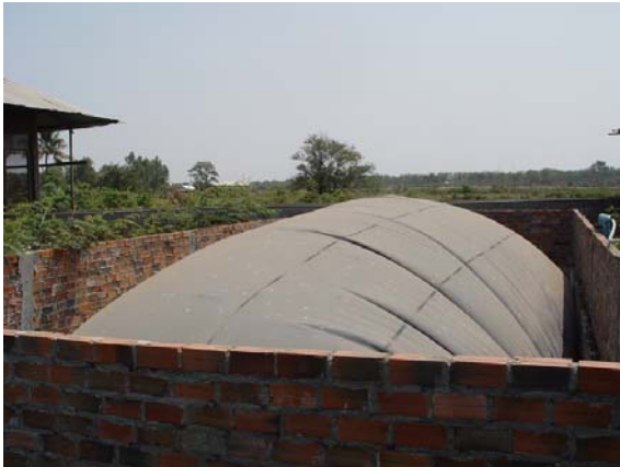
Figure 75: 250 m 3 biogas system at Taing Haing Ly
