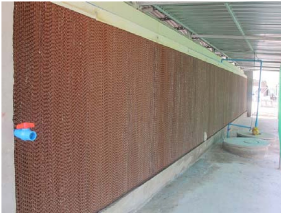
Figure 3: Water curtain of closed stable
