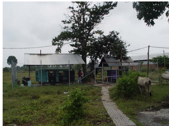
Figure 52: Generators at BVB
