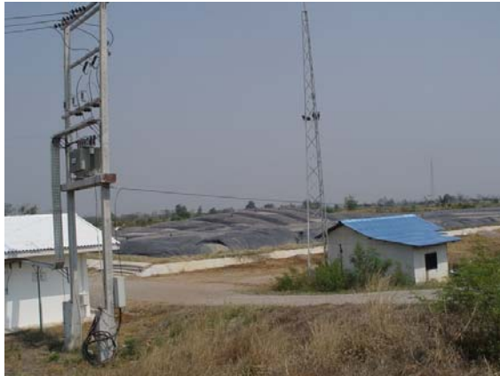
Figure 9: BAI biogas plant
