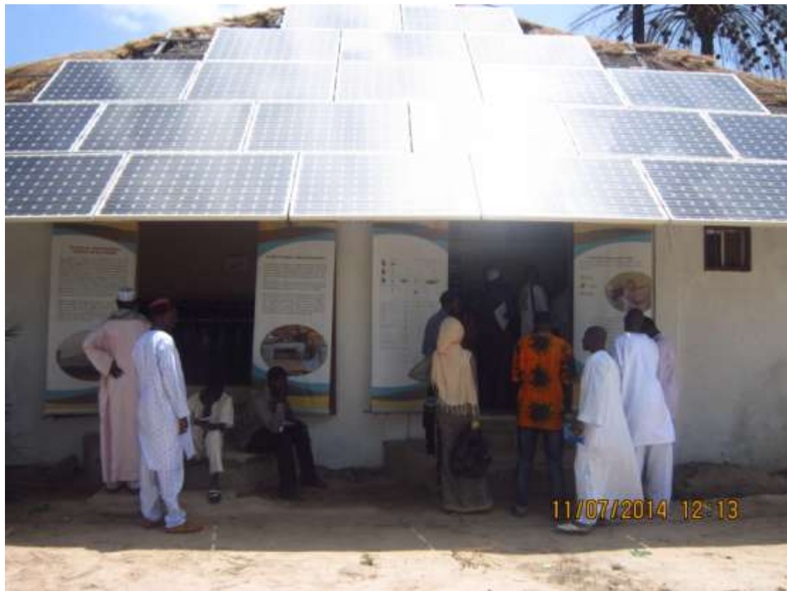
Figure 8 : 6kW off grid solar system at Mbolo
