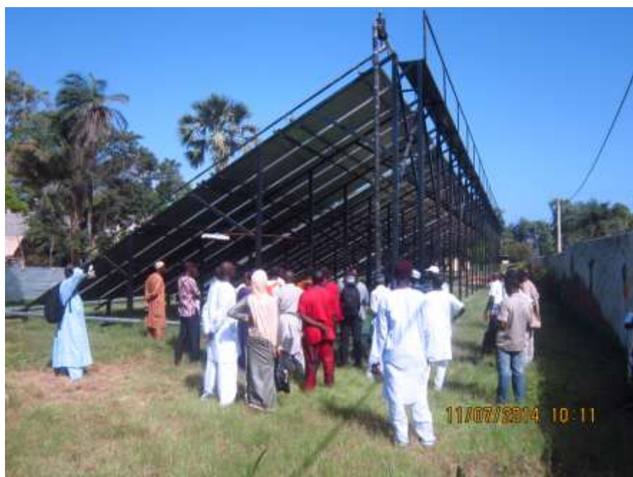
Figure 7 : Participants being shown the installation
