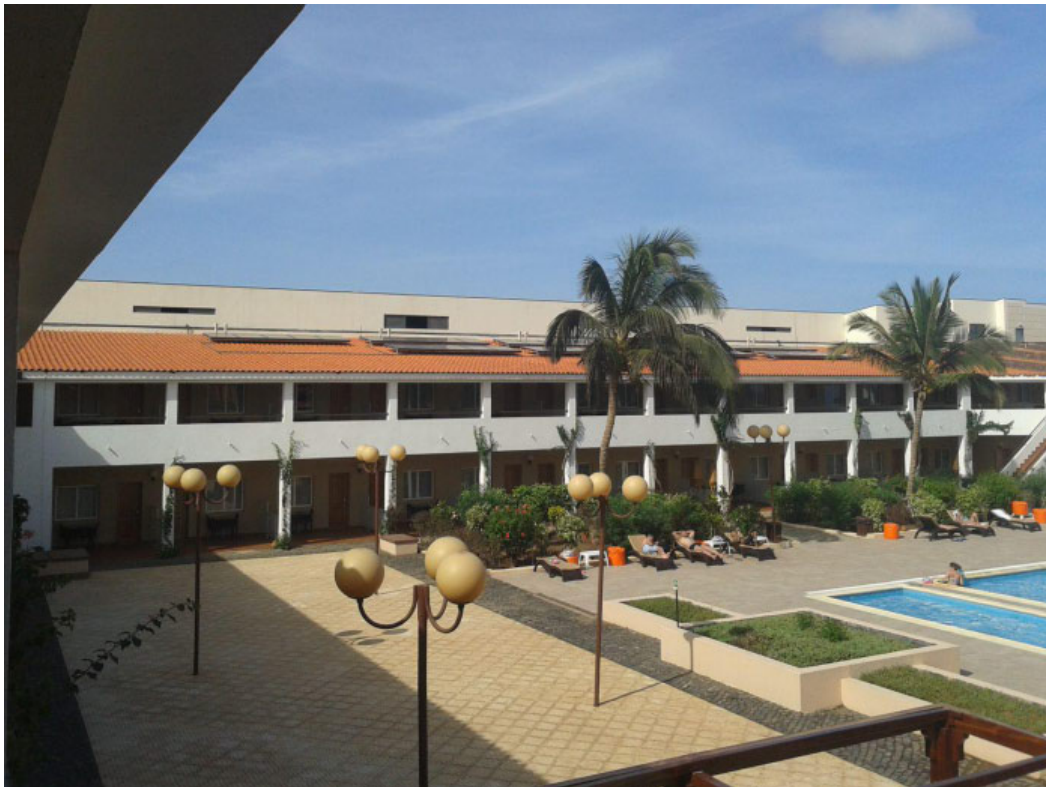
Figure 13: Partial view of PESTANA TRÓPICO Hotel; collectors are roof mounted
