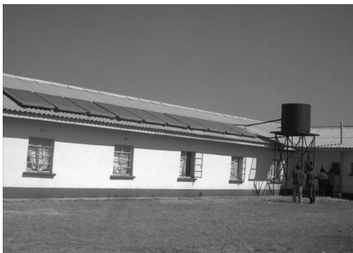
PICTURE 1. LOCALLY PRODUCED THERMOSYPHON SYSTEM FOR A BOARDING SCHOOL, ZIMBABWE.
