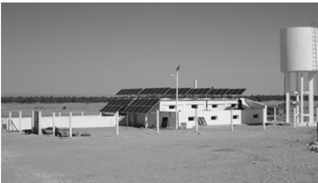
FIGURE 3. THE PV DESALINATION PLANT AT KSAR GHILÈNE (SOURCE: ITC).
