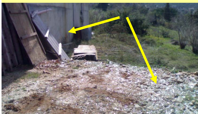
Physical contamination surrounding a food industry in North Lebanon. Note the glass and wreckages beside the main entrance
