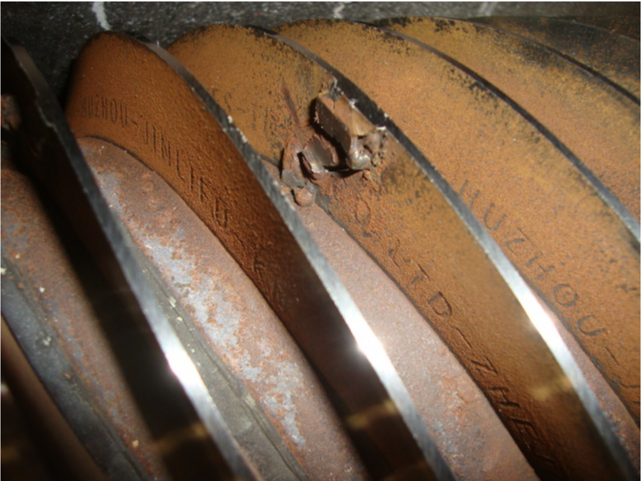
Figure 1 Foreign object used to cover a crack in the blade
