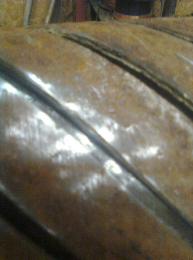
Figure 15 Typical example of damaged and repaired groove
