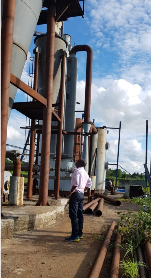
National Evaluation Consultant inspecting the plant
