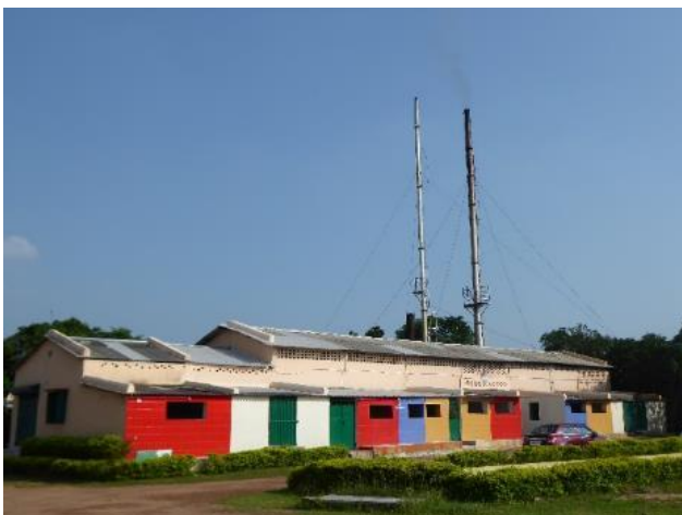
The Sani Clean facility
