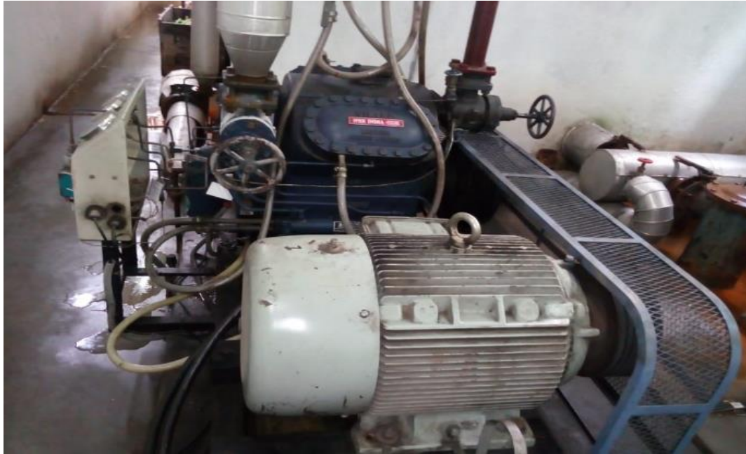
Image 3: Chiller compressor at Sikkim Dairy Cluster
