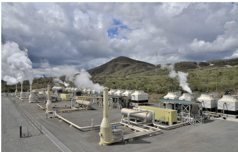
Figure 1: GEG Pilot and Wellhead plants of British Green Energy Geothermal (GEG) at Olkaria, Kenya (source: GEG/Lydur Skulason - https://www.thinkgeoenergy.com/10-years-in-kenya-the-geothermal-success-story-of-geg/ )
