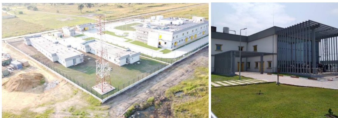
Figure 2: Pictures of the Oyo Centre
