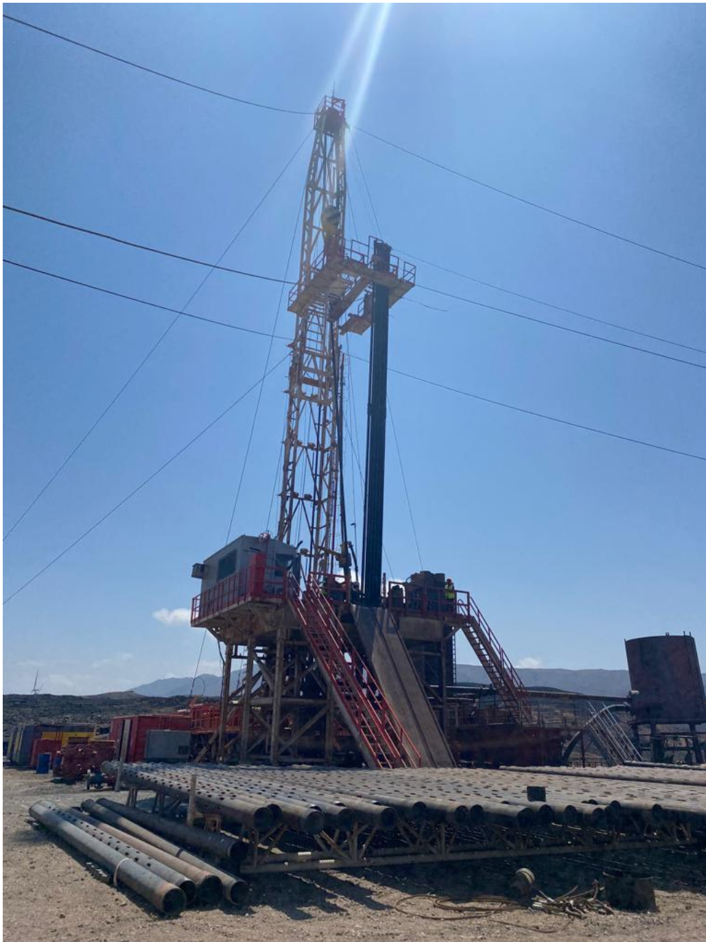
Figure 6: Drilling operation at Gale La Koma in November 2022
