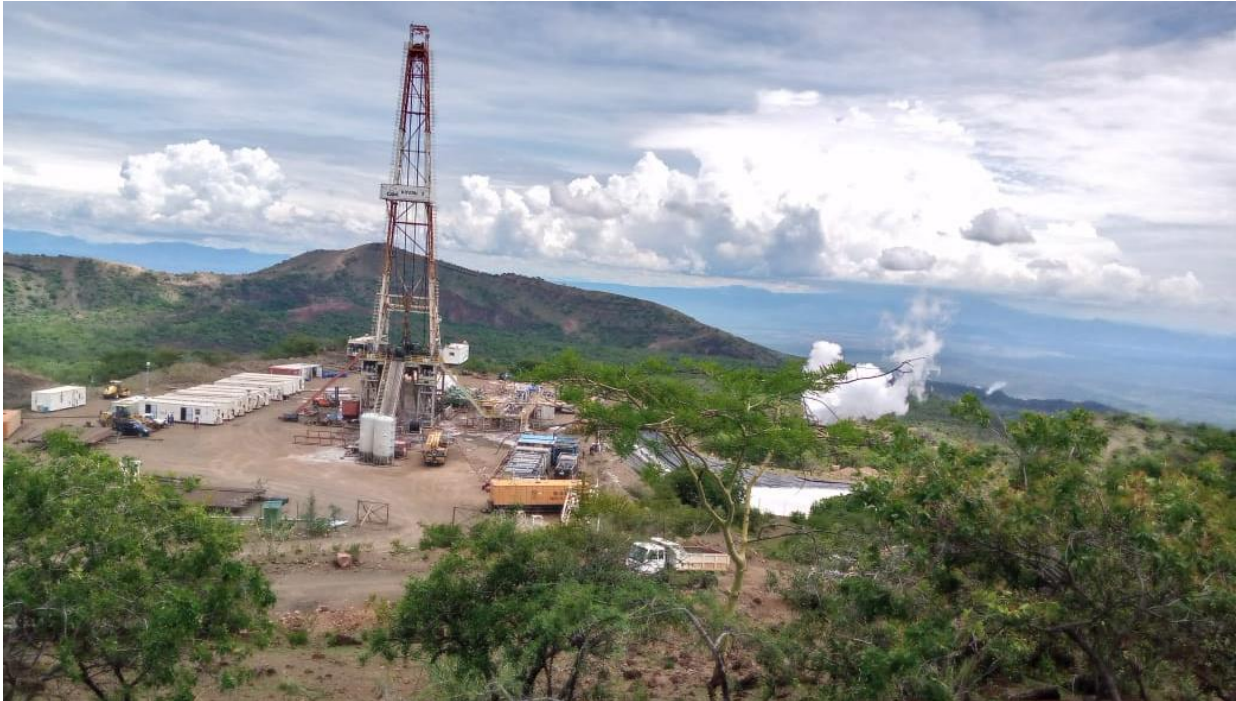
Figure 14: Photo of drilling operations at Paka Geothermal field, Kenya
