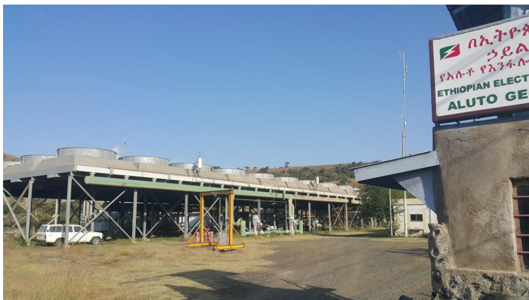
Figure 7: Photo of the 8.5 Aluto Langano 8.5 MW pilot plant commissioned in 1998
