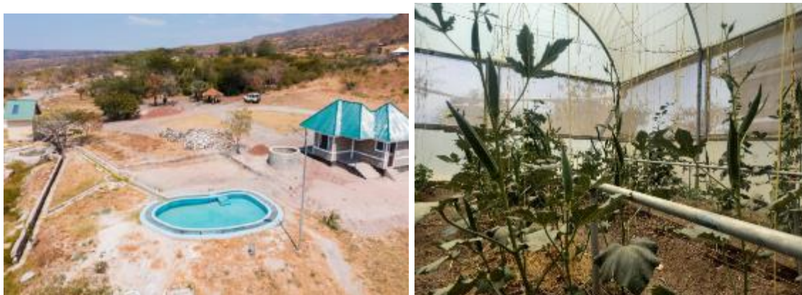
Figure 10: Direct use demonstration facilities at Songwe geothermal area
