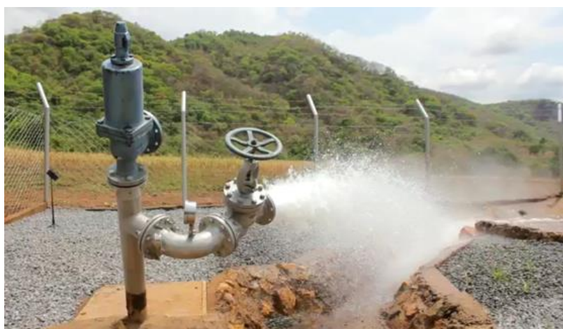
Figure 7: Discharging temperature gradient hole in Mbaka prospect
