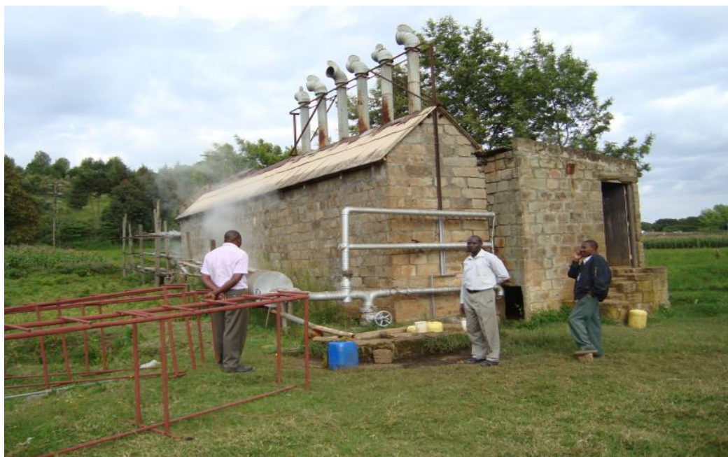
Figure 23: Pyrethrum and grain dryer at Eburru geothermal field
