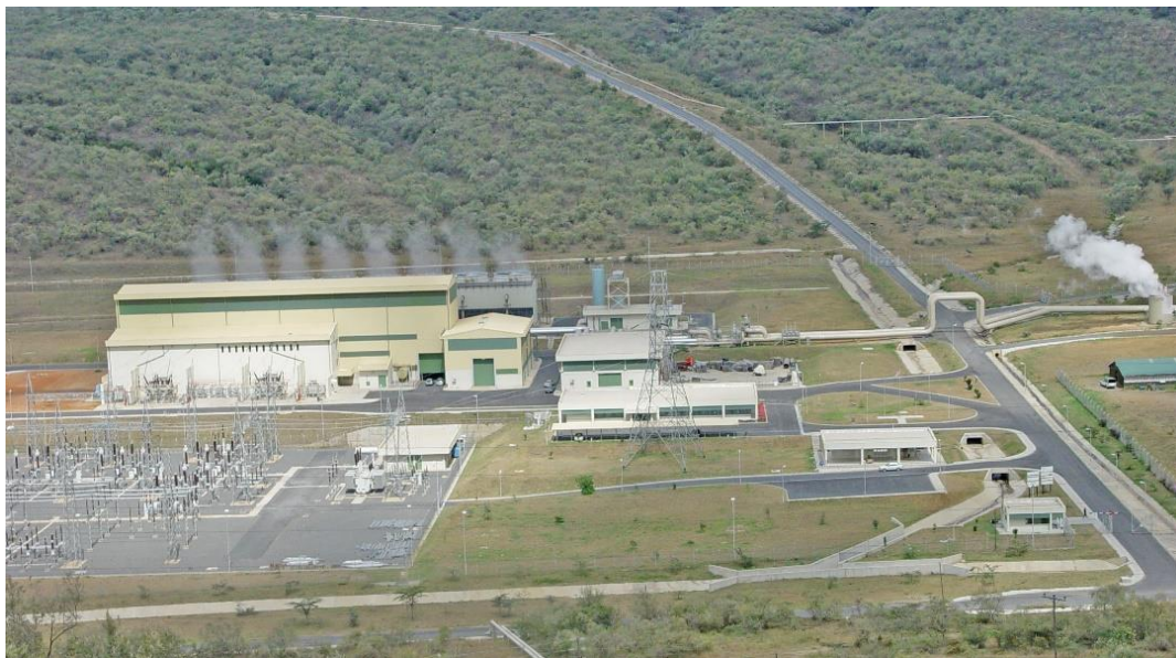
Figure 8: Photo of Olkaria II, 105 MWe Power Plant at Olkaria
