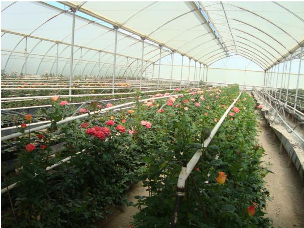
Figure 22: Geothermally heated greenhouse in Kenya. The white pipes carry hot water
