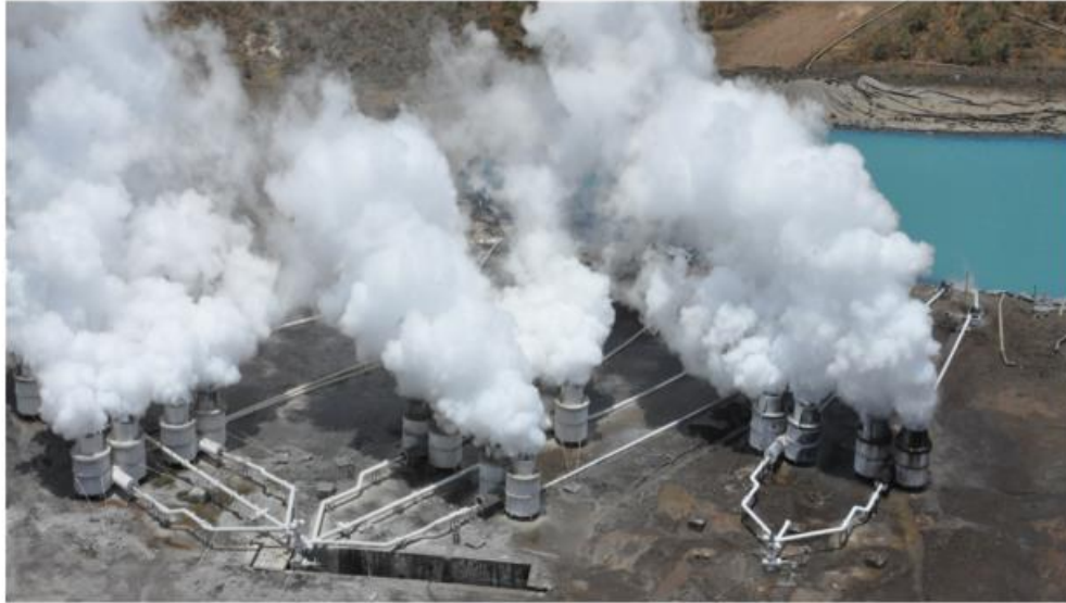
Figure 17: Discharge testing of Menengai well MW-01A producing 30MWe.
