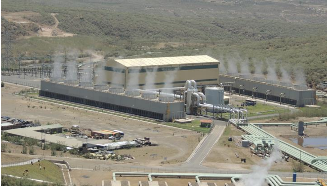
Figure 9: Photo of Olkaria IV, 150MWe Power plant
