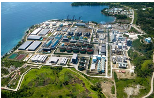
The Papua New Guinea Ruimu Nickel and Cobalt Project applied China ENFI’s independently developed high pressure acid leaching-nickel-cobalt precipitation technology
