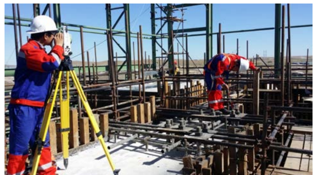
Precise positioning of pre-embedded bolts
